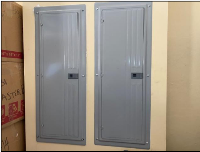
58. The home inspector shall observe: Service...
