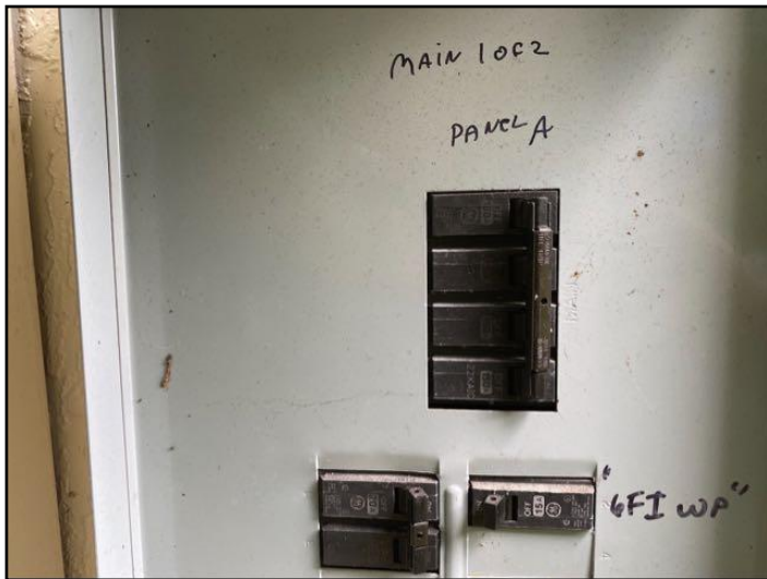
53. The home inspector shall observe: Service...
