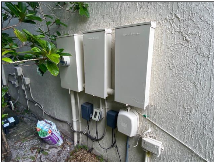
52. The home inspector shall observe: Service...
