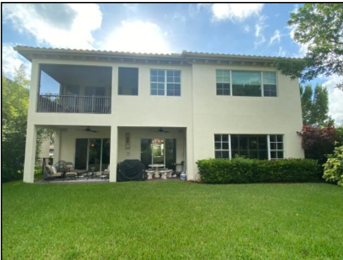
25. The home inspector shall observe: Wall...
