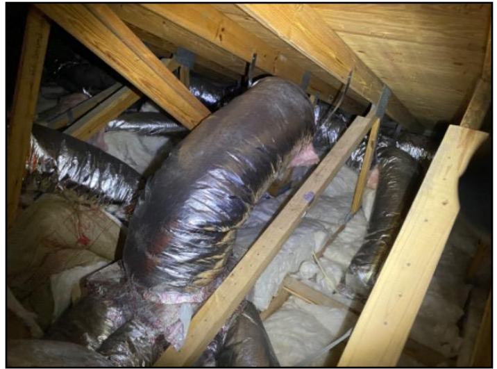
47. The home inspector shall observe: Wall...
