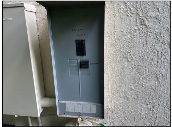
55. The home inspector shall observe: Service...
