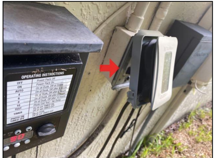
83. The home inspector shall observe: Service...
