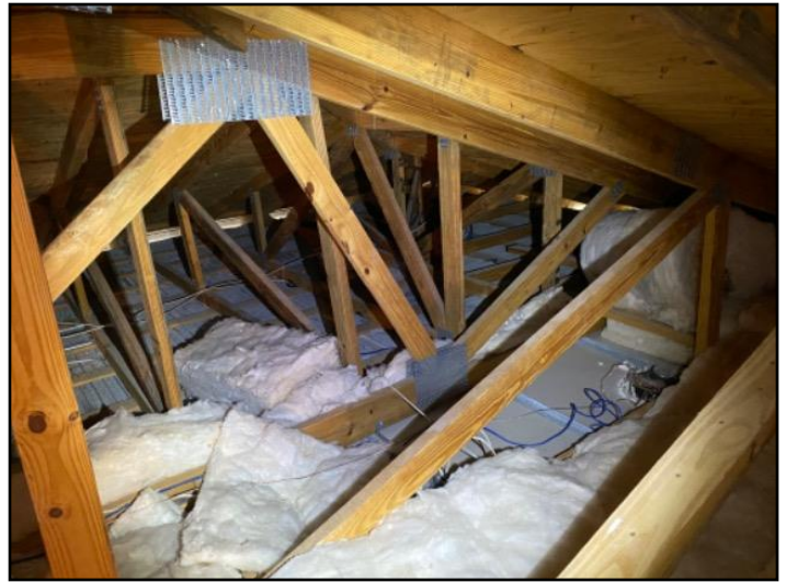
43. The home inspector shall observe: Wall...
