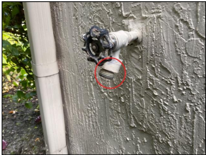
146. Backflow prevention missing
