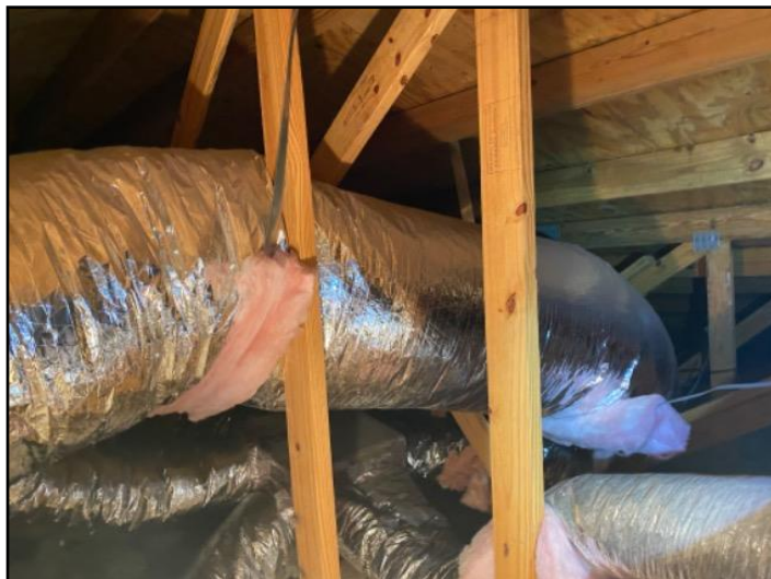
41. The home inspector shall observe: Wall...
