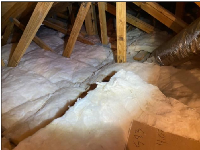
40. The home inspector shall observe: Wall...
