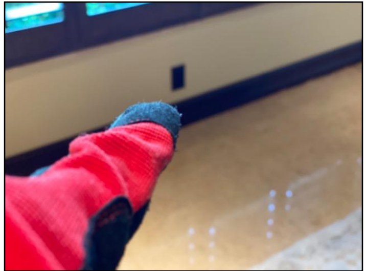
75. 1st Floor Outlet - Westside
