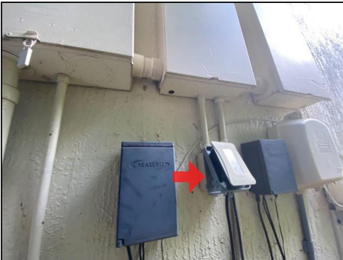
82. The home inspector shall observe: Service...
