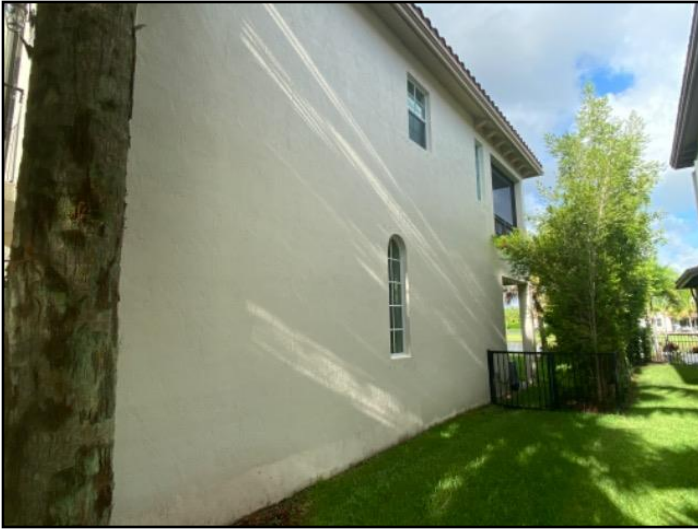
23. The home inspector shall observe: Wall...
