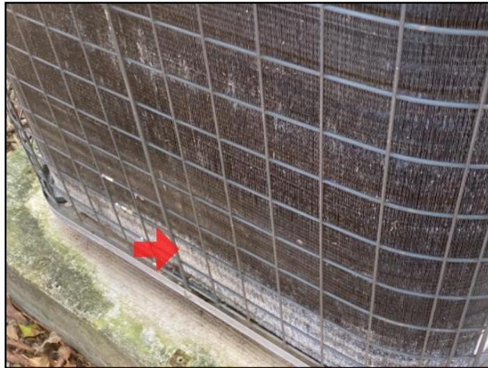
102. Service air conditioner
