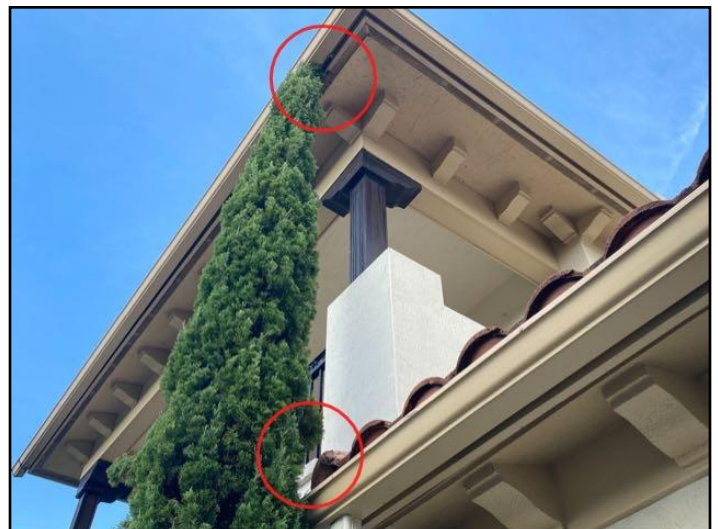
37. The home inspector shall observe: Wall...
