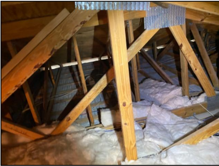
42. The home inspector shall observe: Wall...
