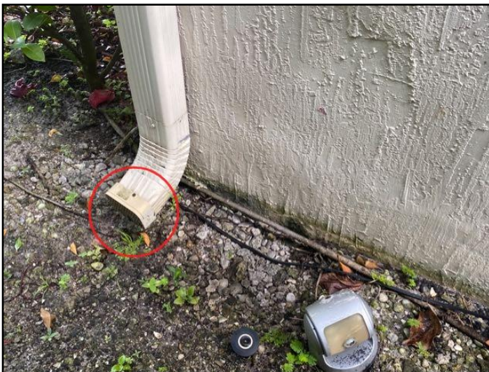
34. The home inspector shall observe: Wall...
