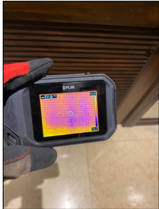
99. 77° - Return Temp (1st Flr)
