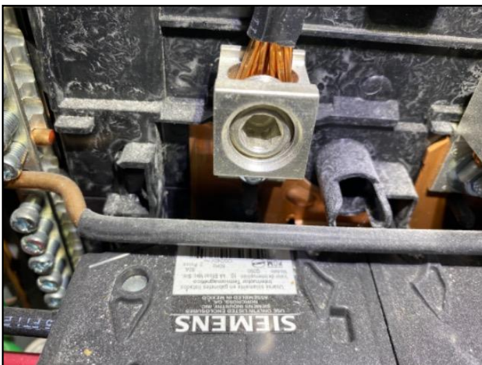
72. The home inspector shall observe: Service...
