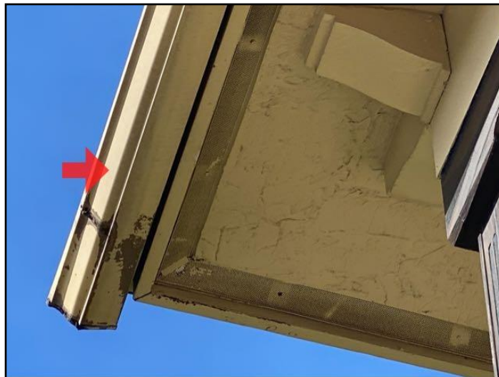
28. The home inspector shall observe: Wall...
