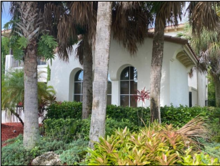
21. The home inspector shall observe: Wall...
