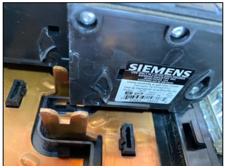
69. The home inspector shall observe: Service...
