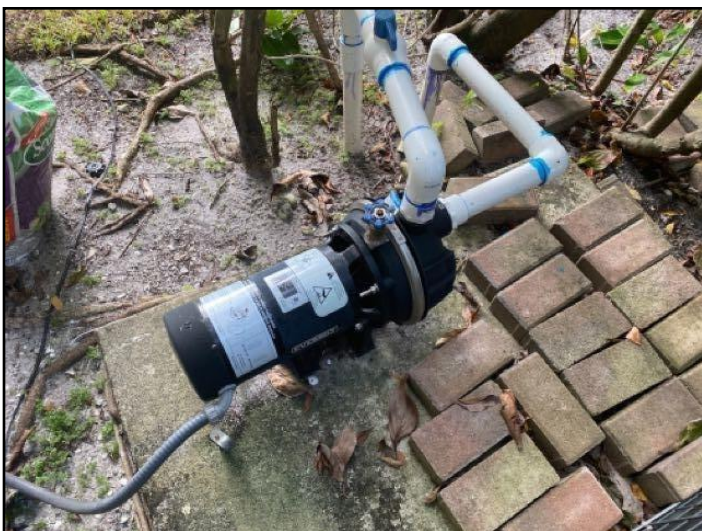
139. Landscape irrigation system
