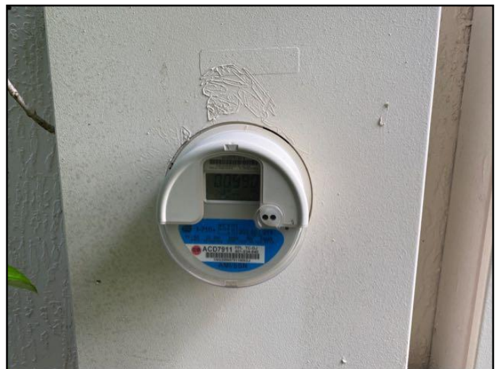
57. The home inspector shall observe: Service...
