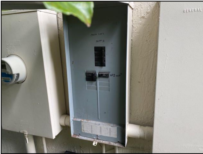
54. The home inspector shall observe: Service...
