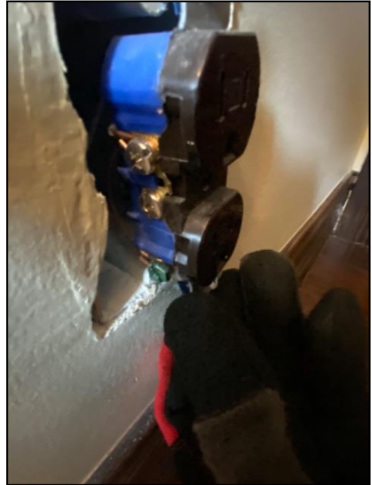
79. 2nd Floor Outlet - Eastside
