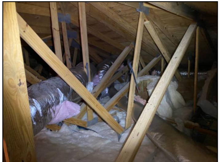
45. The home inspector shall observe: Wall...
