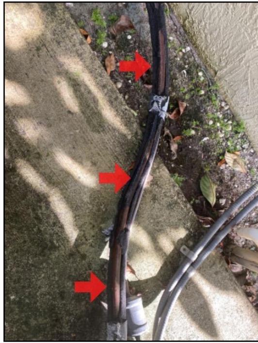
118. Insulation - missing
