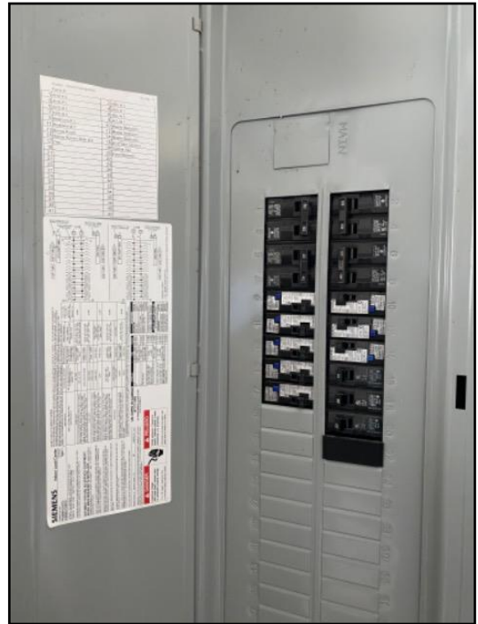
59. The home inspector shall observe: Service...
