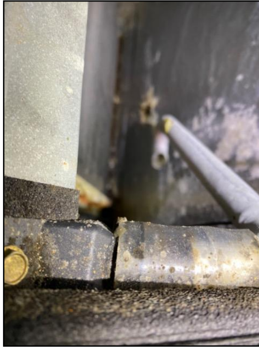
116. Service air conditioner
