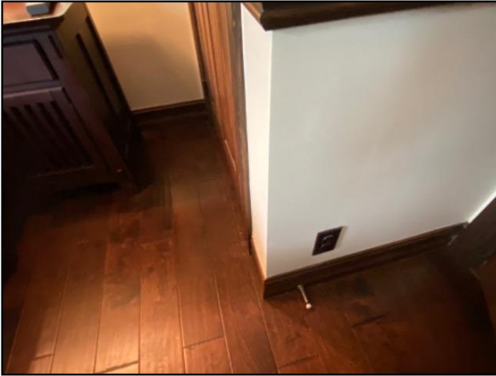
78. 2nd Floor Outlet - Eastside
