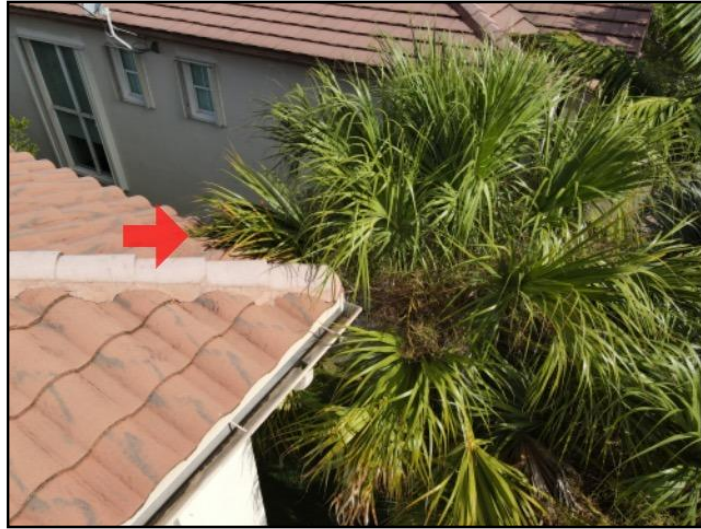
38. Trees or shrubs too close to building
