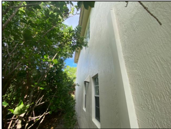
27. The home inspector shall observe: Wall...
