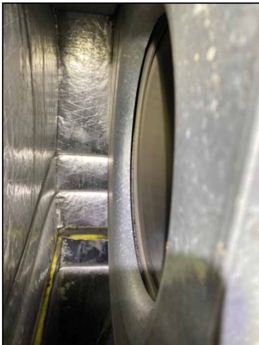
114. Service air conditioner
