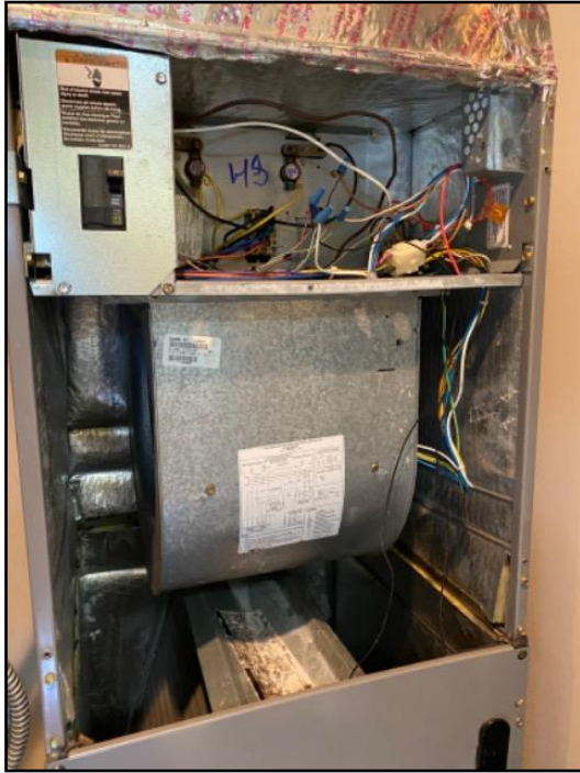
108. Service air conditioner
