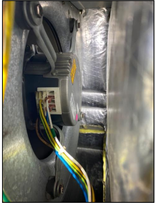
113. Service air conditioner
