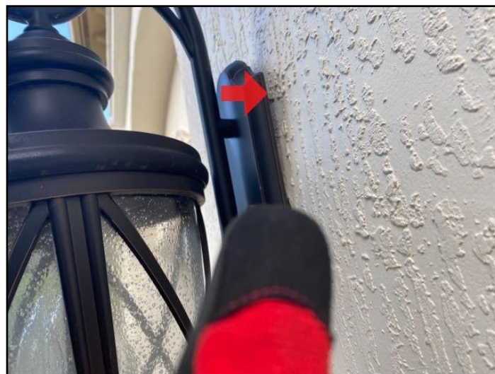
85. The home inspector shall observe: Service...
