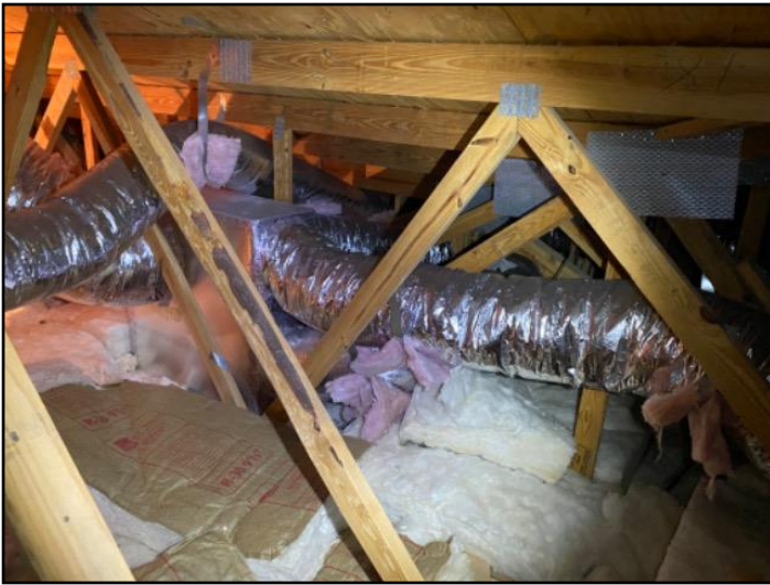
46. The home inspector shall observe: Wall...
