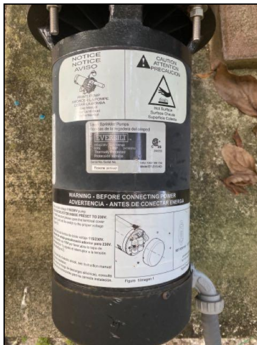
140. Landscape irrigation system
