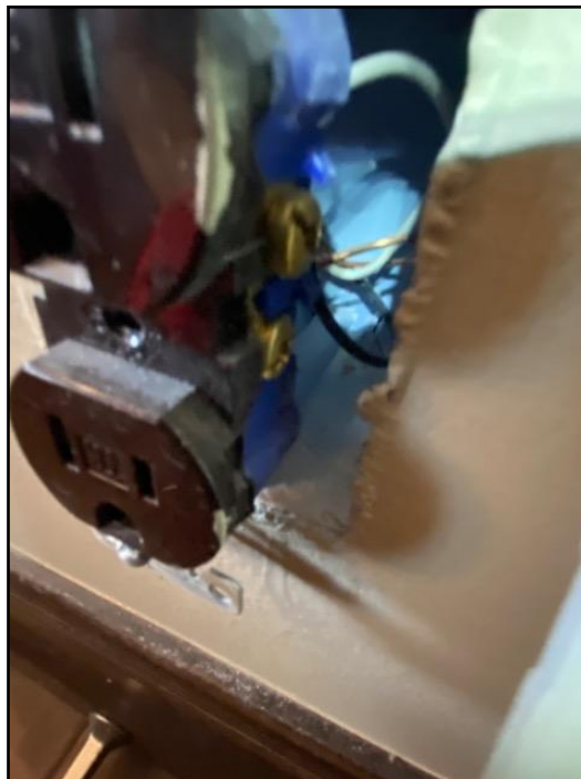
80. 1st Floor Outlet - Westside
