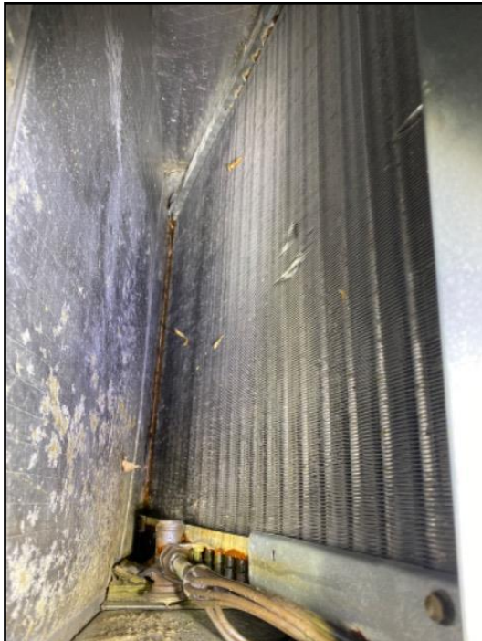
110. Service air conditioner
