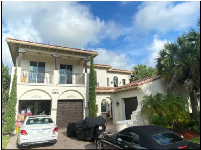
22. The home inspector shall observe: Wall...
