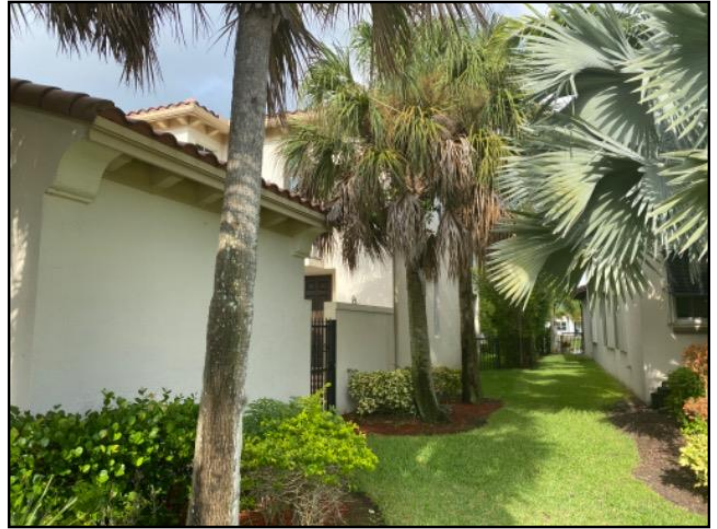
24. The home inspector shall observe: Wall...
