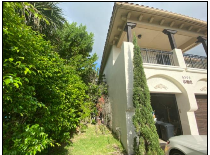
26. The home inspector shall observe: Wall...
