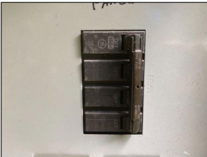
56. The home inspector shall observe: Service...
