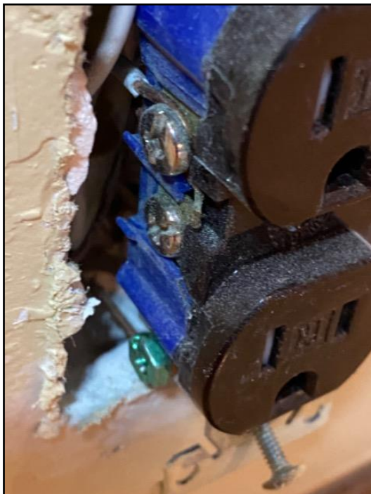
76. 2nd Floor Outlet - Eastside
