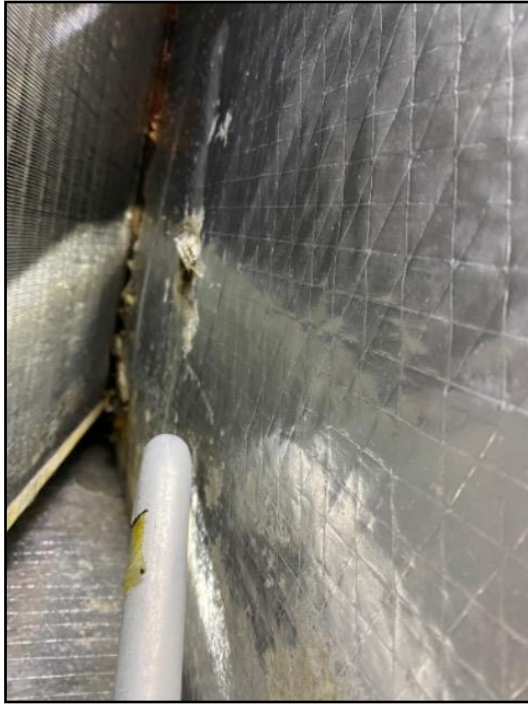
112. Service air conditioner
