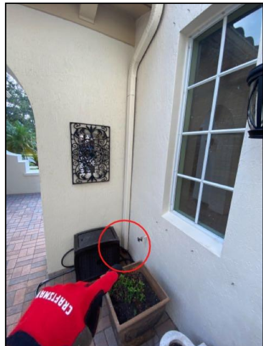
35. The home inspector shall observe: Wall...
