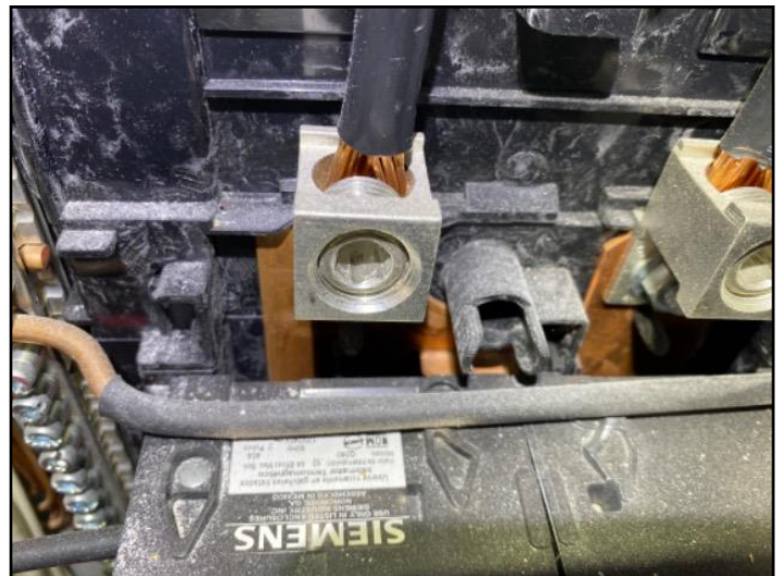
65. The home inspector shall observe: Service...
