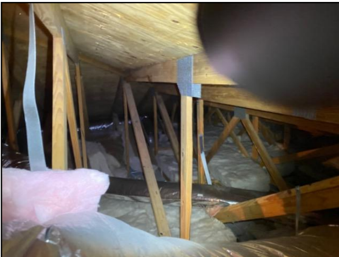
44. The home inspector shall observe: Wall...
