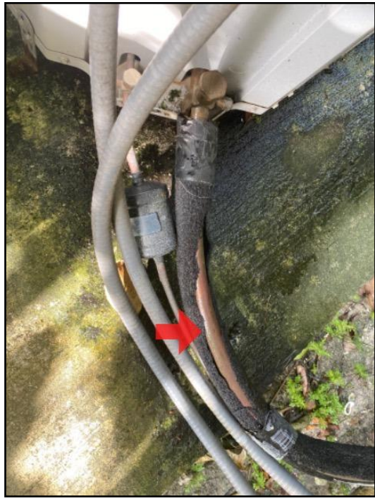
117. Insulation - missing
