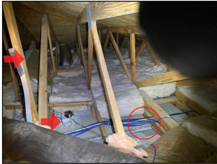
122. Gaps or voids
