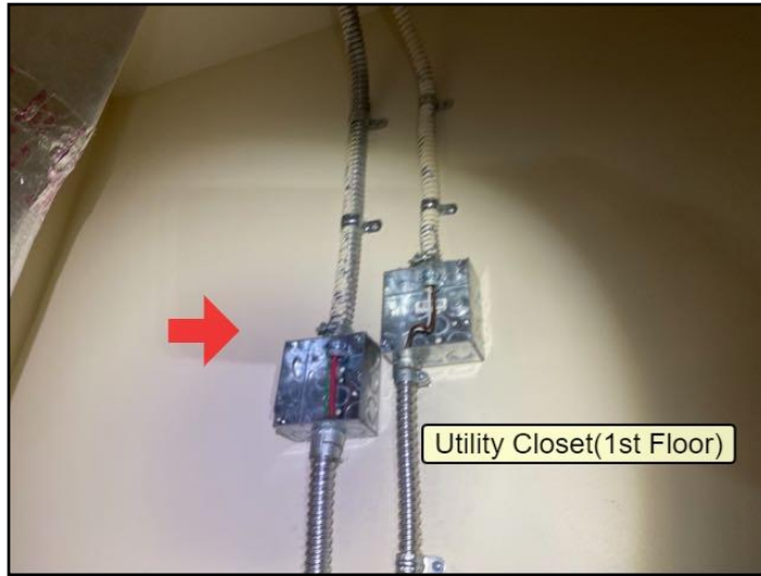
81. The home inspector shall observe: Service...
