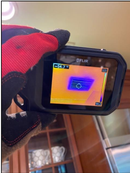
98. 55° - Supply Temp (1st Flr)
