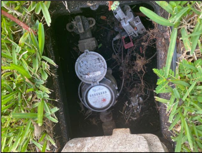
125. Main Water Valve
