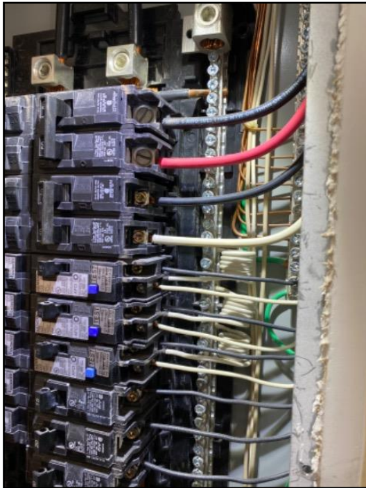
74. The home inspector shall observe: Service...
