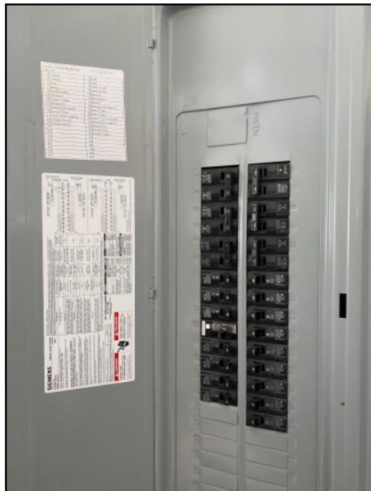
60. The home inspector shall observe: Service...
