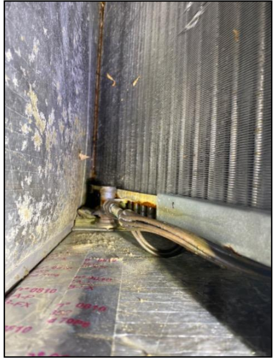
109. Service air conditioner
