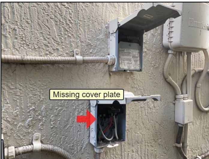
87. Service Disconnects Present
