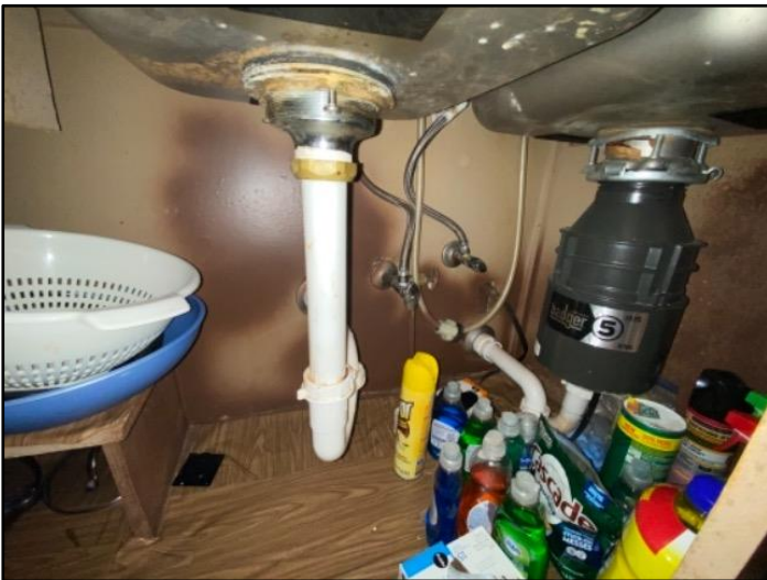
Under the Kitchen Sink
