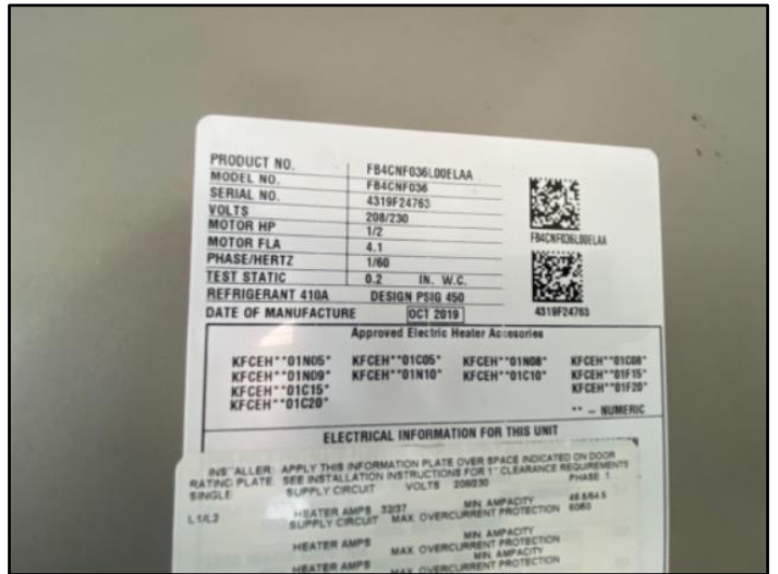
Air Handler Label
