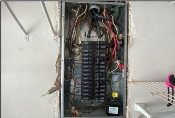
Electrical Panel Cover removed
