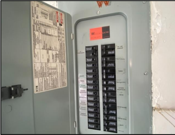
Electrical Panel and Label
